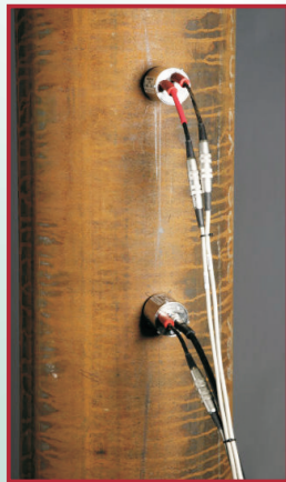
Online coal mass flow sensors installed on a coal pipe.
